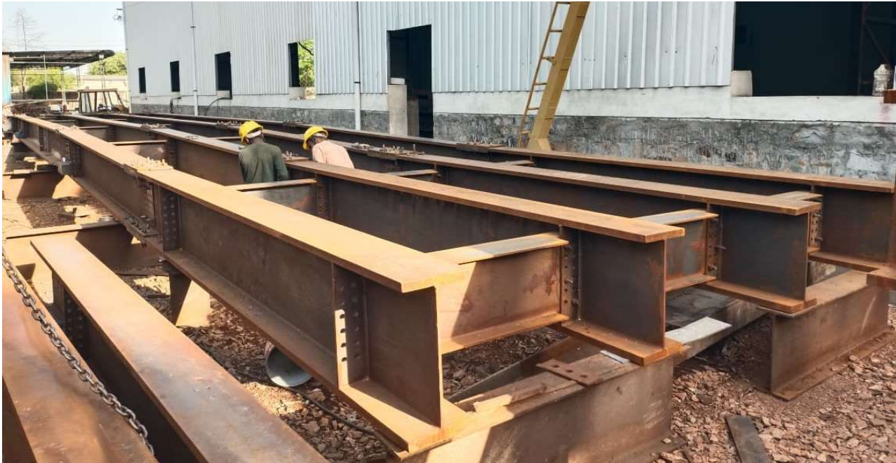
FOB GIRDER : MAVLI STATION
