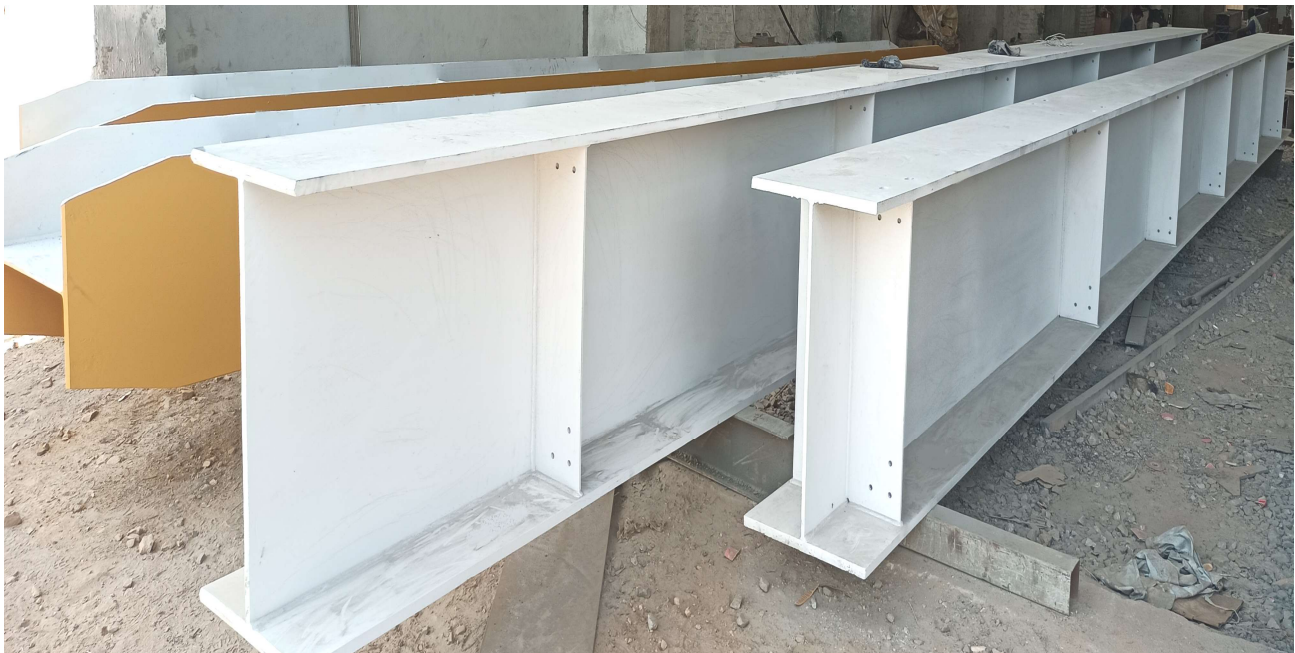
FOB GIRDER : BAYANA STATION CONTRACTOR: M/S. KRISHNA PAL SINGH KANPUR
